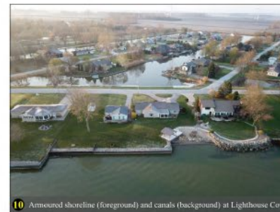
10 Armoured shoreline (foreground) and canals (background) at Lighthouse Cove.
