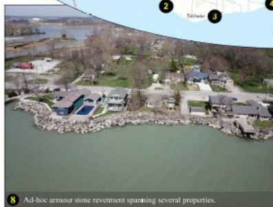
8 Ad-hoc armour stone revetment spanning several properties.
