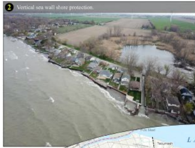
2 Vertical sea-wall shore protection.
