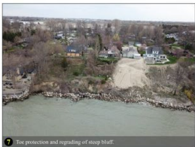
7 Toe protection and regrading of steep bluff.
