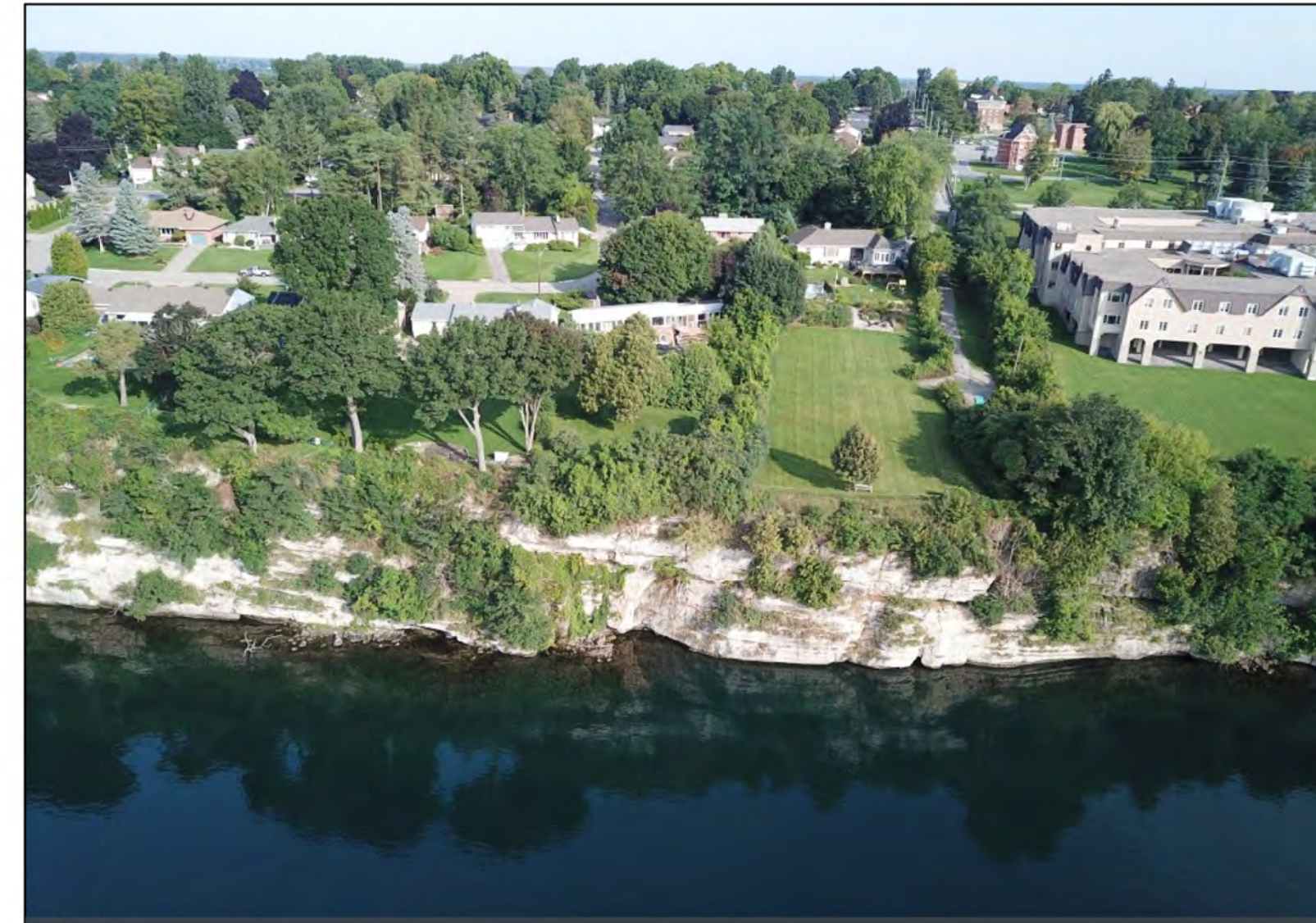
10 Vertical bedrock cliffs.
