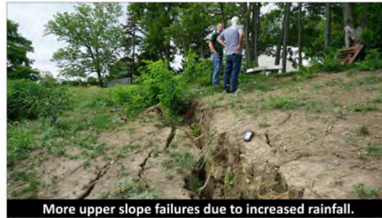
More upper slope failures due to increased rainfall.
