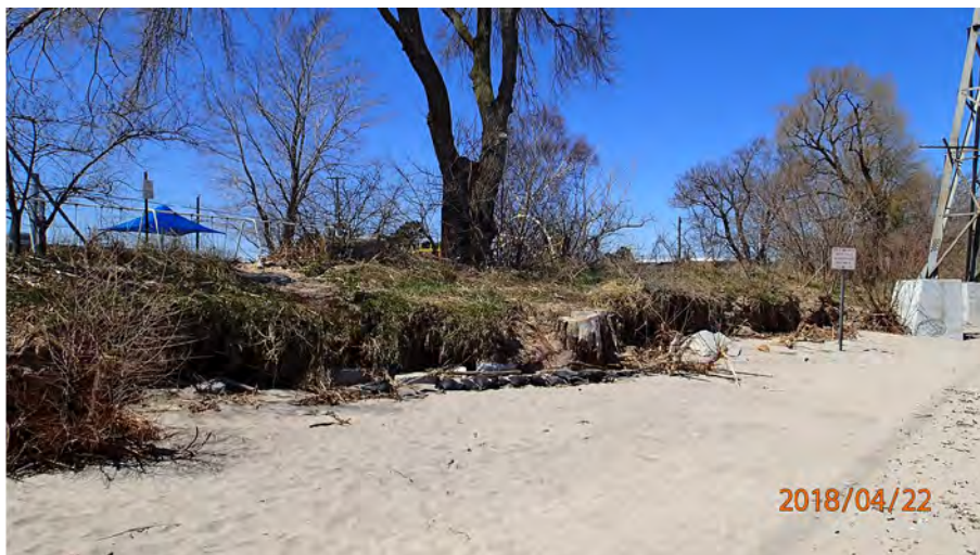
Figure 2.6 Eroded Dune at Parkette
