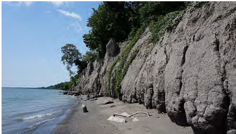
Figure 2.24 Eroding Bluffs in Region 1E
