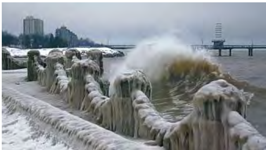
Figure 2.3 Ice-covered Seawall at Spencer Smith Park
