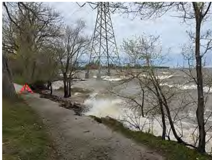
Figure 2.1 Erosion of Trail during 2017 High Lake Level Conditions
