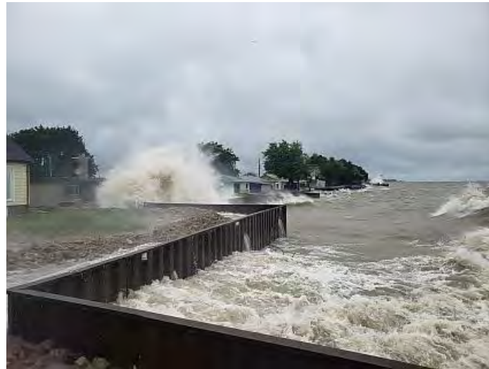
Figure 2.31 Direct Wave Attack on Buildings, August 27, 2019 Storm
