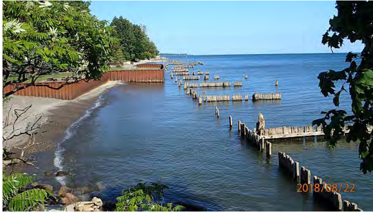
Figure 2.28 Old Timber Groynes and New Steel Sheet Pile Wall (2018.08.22)
