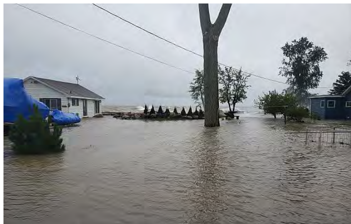
Figure 2.30 Flooding of Building Foundations, August 27, 2019 Storm
