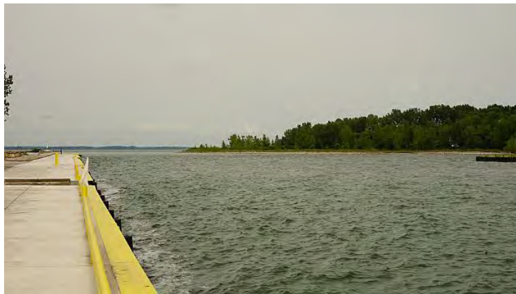
Figure 2.40 Navigation Channel Looking into Rondeau Bay
