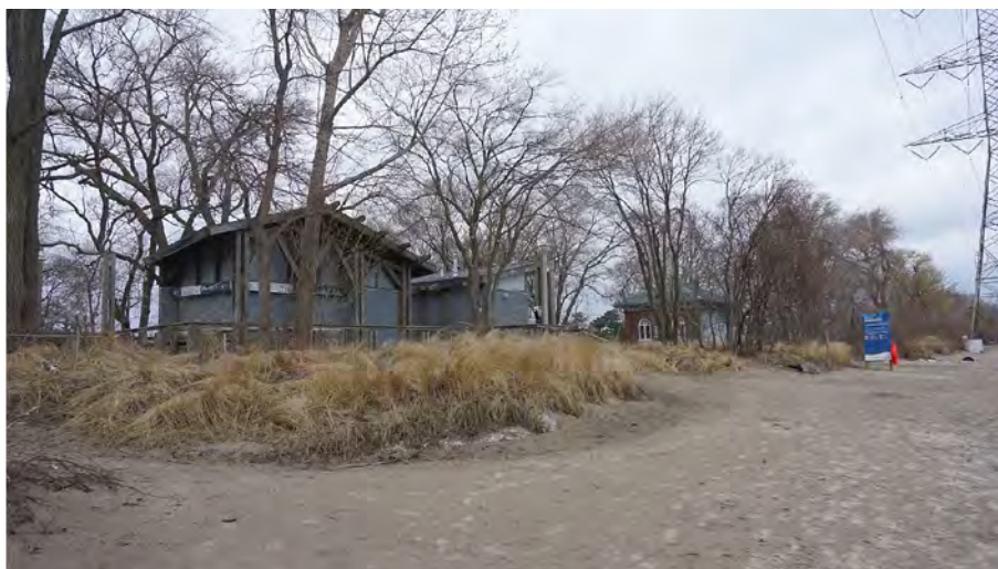
Figure 2.8 March 15, 2019 Conditions at the Pavilion
