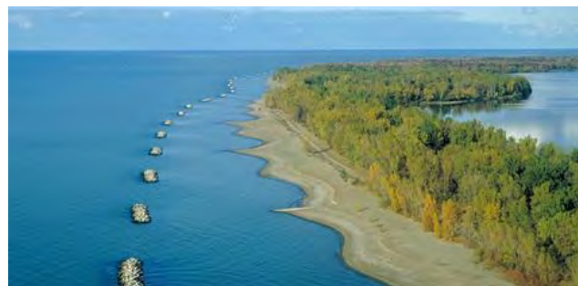
Figure 6.8 Offshore Breakwaters Presque Isle State Park, Pennsylvania
