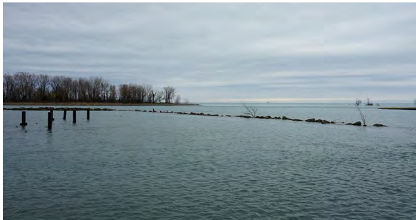
Figure 6.26 Crest of the Fishing Fleet Breakwater in May 2019 (crest almost submerged)
