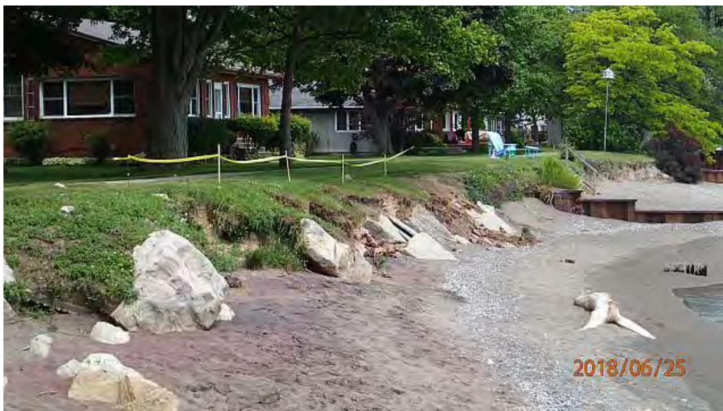
Figure 2.27 Erosion of the Backshore between the Groynes at Erie Beach
