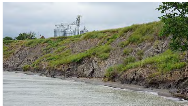
Figure 2.17 Port Alma Bluffs on August 22, 2018 (same location as Figure 2.16)
