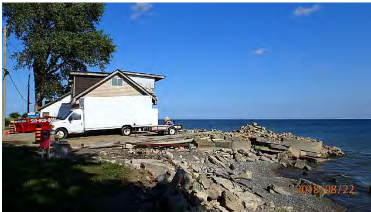
Figure 2.29 Dumped Concrete Rubble Shore Protection (2018.08.22)
