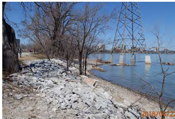
Figure 2.2 Re-alignment of the Trail and Shoreline Armouring in 2018
