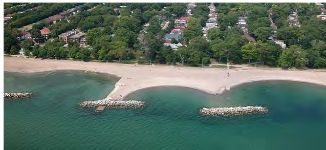
Figure 6.7 Offshore Breakwaters Eastern Beaches, Toronto
