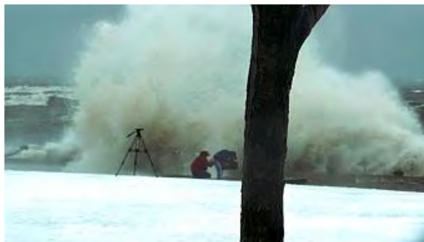
Figure 2.4 Wave Overtopping at Spencer Smith Park
