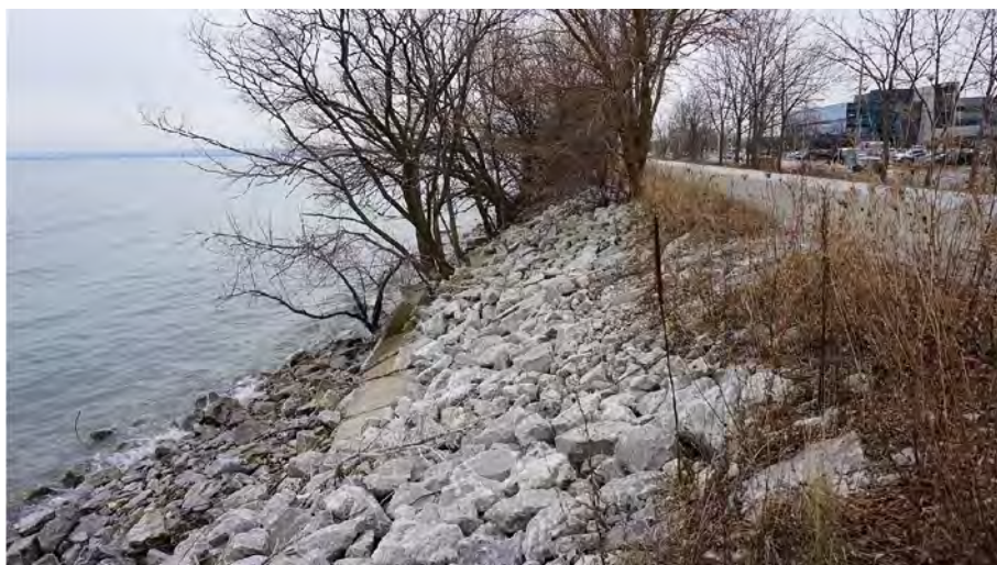
Figure 2.16 Armoured Slope along the Living Shoreline
