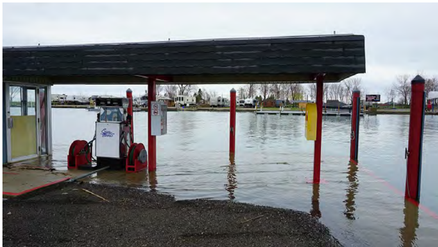
Figure 6.24 Submerged Fuel Dock in Erieau, May 7, 2019
